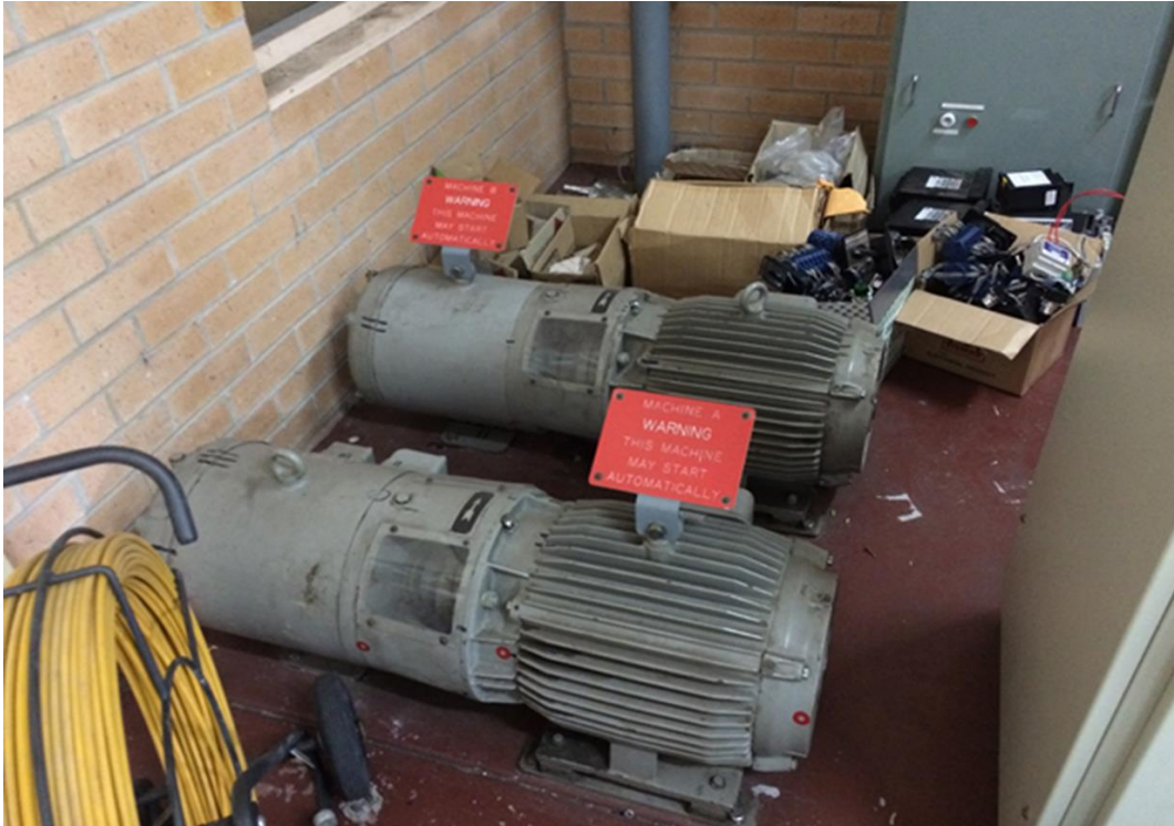
Figure 1 - AFIC MG (Motor Generator) set
